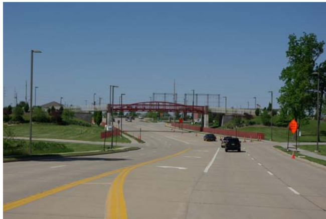
T.R. Hughes Boulevard at T.R. Hughes Ballpark pedestrian bridge.
