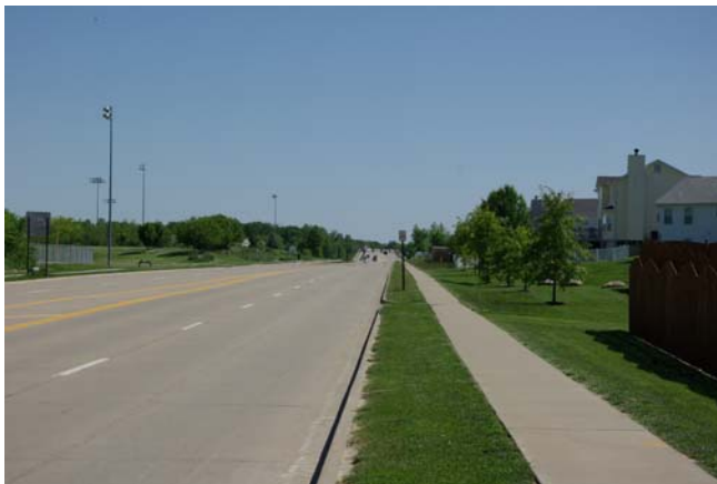
T.R. Hughes Boulevard looking south towards bridge over railroad and creek.
