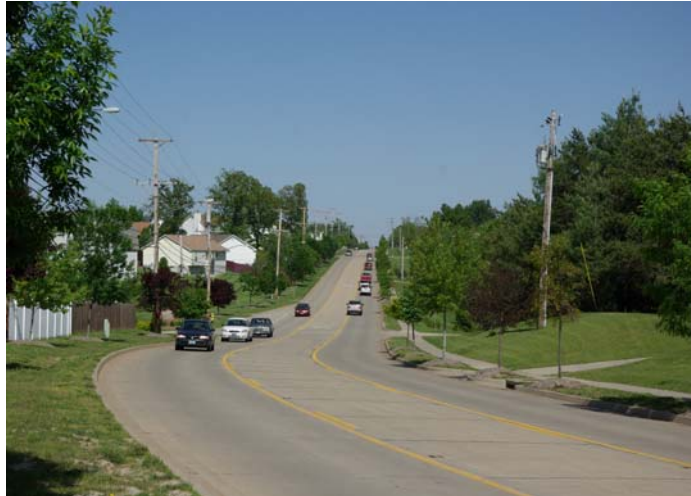
Feise Road – looking east along new alignment.
