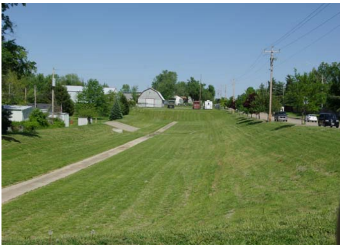
Feise Road – stormwater detention facility.
