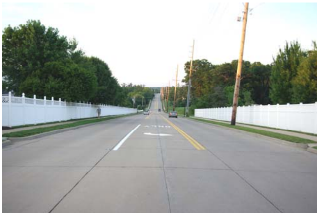
Hackmann Road looking east towards Muegge Road.
