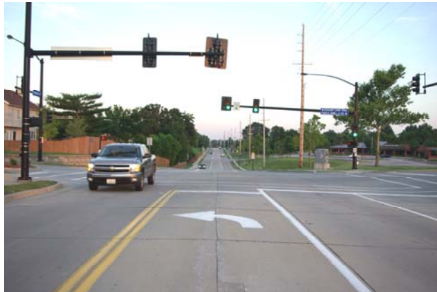
Hackmann Road at the entrance to Francis Howell North High School.
